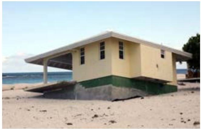
Damaged beach villa on Anegada, BVI. Sandbags trying to support beach nourishment are visible (photo: Ilan Kelman).
