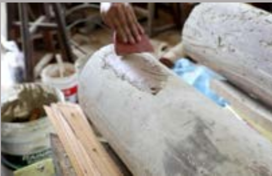
Restoration of the pillar of "dharma rain and luminous spirits" in Tien Jyun Temple of Chenggong Community: layering with pig's blood-lime mortar (jhu siě huei).
